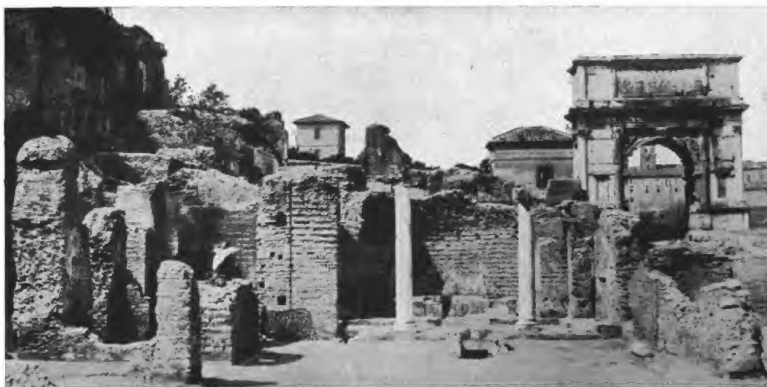
Fig. 211 — S. Maria de Metrio. General view of the apse (from SOPRINTENDENZA, op. cit. ).
